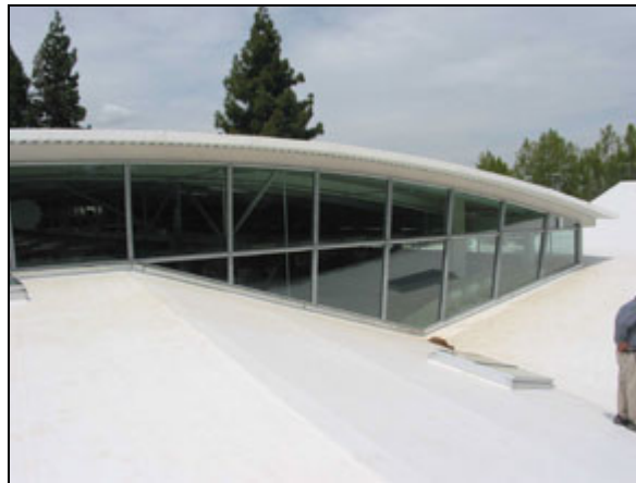
Figure 6.2: Example of a cool roof (fypower.org).
